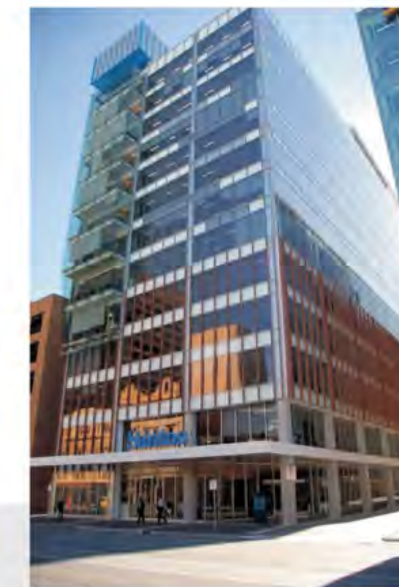
Building height reduced by 10 ft to comply with town planning requirements
